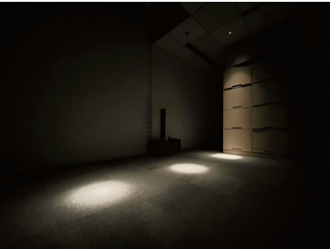
Demonstration of DD130-7° (3.5W) at 2.5 meter ceiling height
